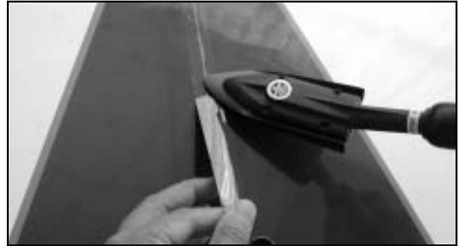
□ Iron the enclosed Trim Tape at the wing joint.
